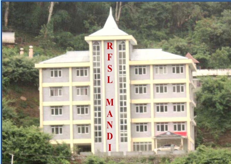
A Complex of RFSL, CR, Mandi (Front View)
